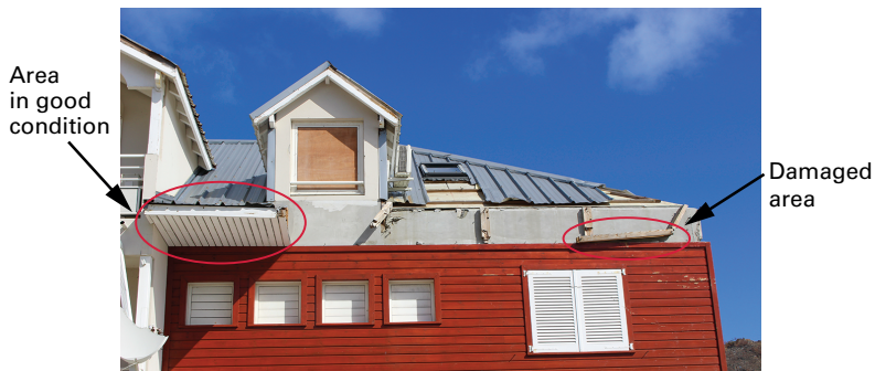
Figure 4: Undersized eave
