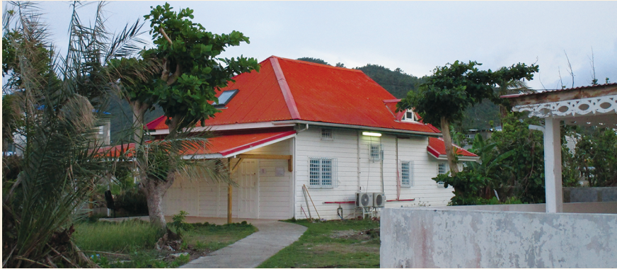
Figure 1: Roof that withstood
