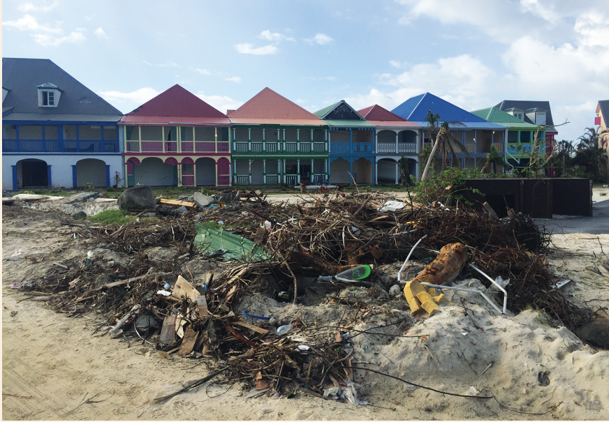
Figure 1: Exposed structure that survived
