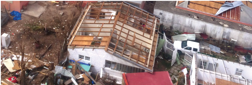
Figure 4: No bracing
