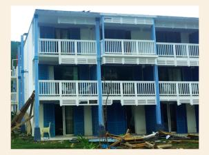
Figure 2: Louvred shutters that provided good protection
