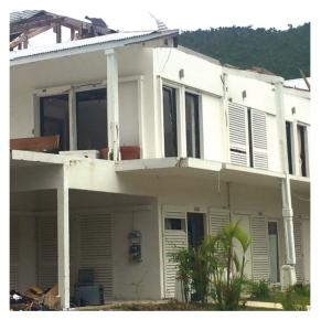
Figure 3: Insufficiently-attached shutters
