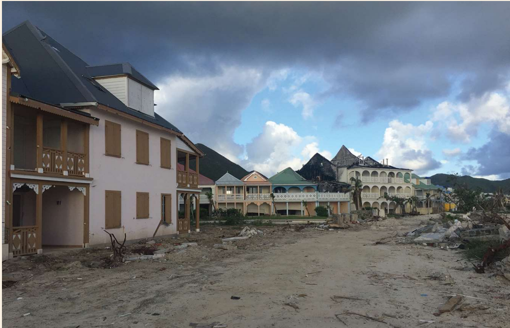
Figure 1: Exposed structures that survived
