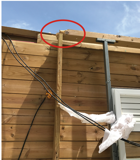
Figure 1: Cross-section probably not substantial enough (CAUE)
