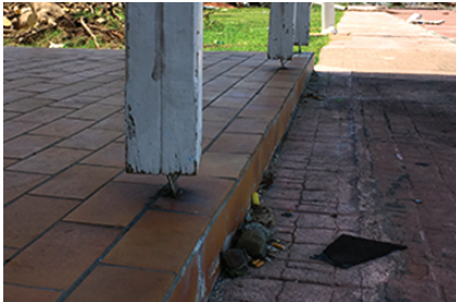
Figure 5: Post base bending
